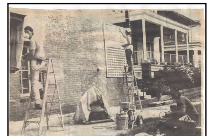
1989 Repairs to Brady Craig
