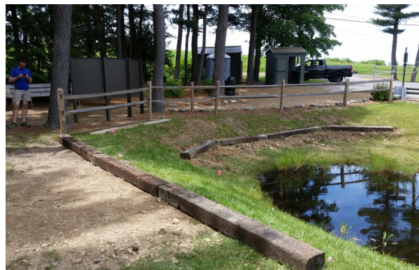
Terracing of the pond area begins.
