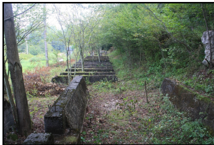
Concrete piers that supported the machinery and sand storage bins inside the 190 foot long and 40 foot wide sand
