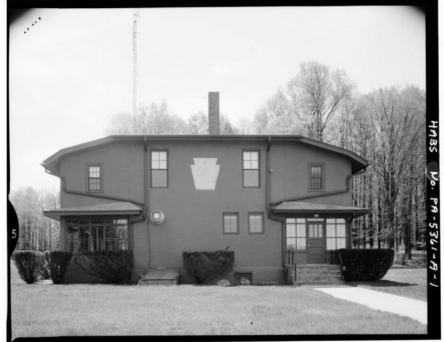
This view of the north entrance to the PA Game Commission's original School of Conservation
